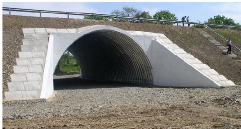
Figure 1. Picture of a Soil-Steel Bridge (Source:www.armtec.com)
