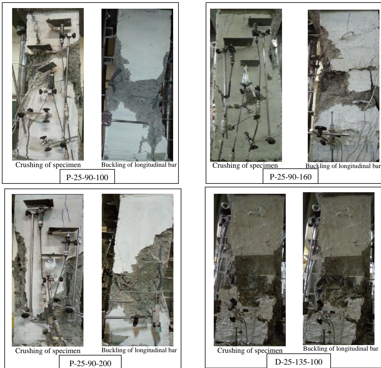
Figure 3. Modes of failure of specimens 1,2,3 and 4
