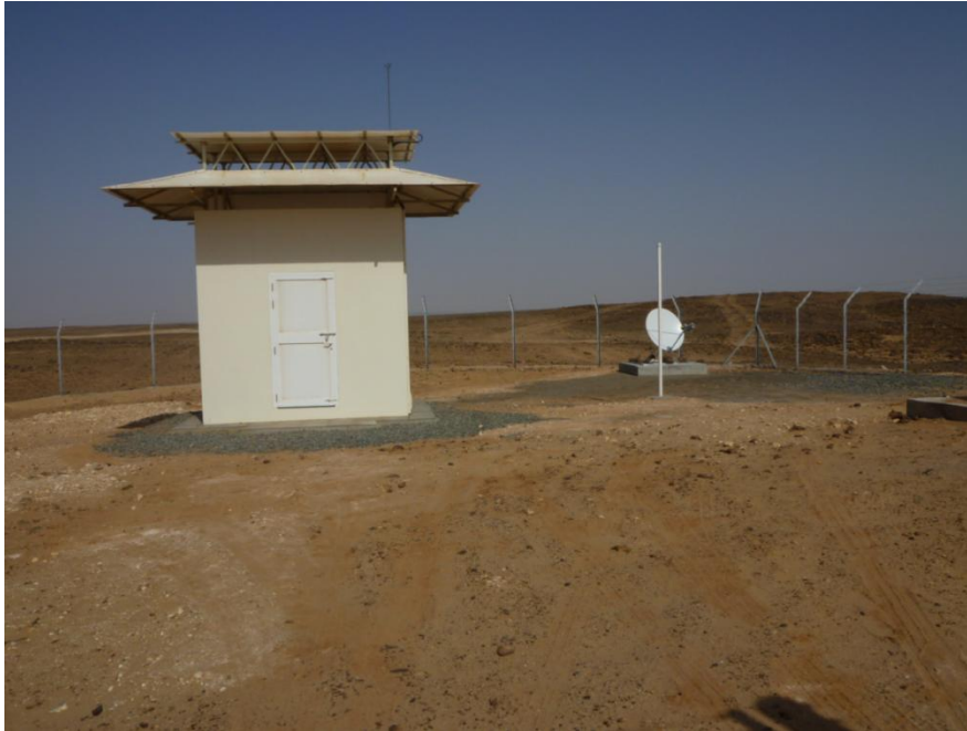
Figure 7. General view of remote station.
