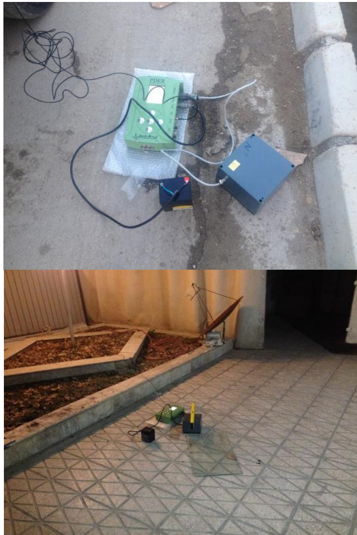
Figure 4. The stations installed in the city.
