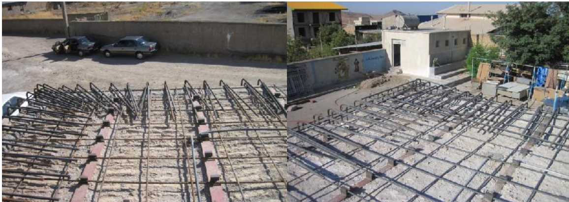
Figure 6. Sample pictures of retrofitting roofs
