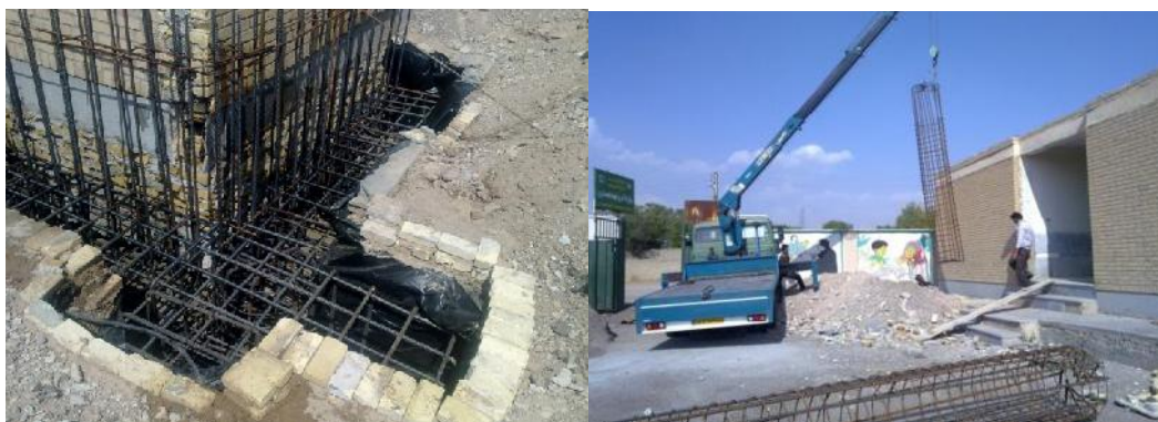
Figure 11. Sample pictures of piles
