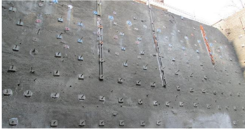
Figure 1. Soil nail wall of the present study
