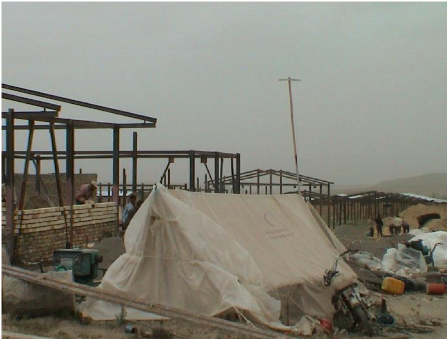
Figure 1. Emergency shelter in Avaj earthquake
