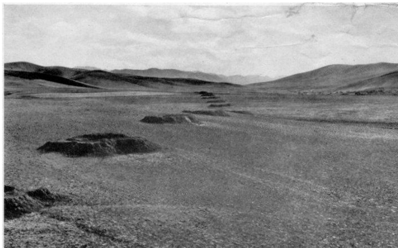
Figure 2. Example of a line of circular craters. Spoil from the excavation of the qanat, and from subsequent periods of maintenance, is piled around the vertical access shafts to provide a wall to protect the shafts and the tunnel below from erosional damage from the inflow of water during a heavy desert rainstorm (Wulff, 1968).
