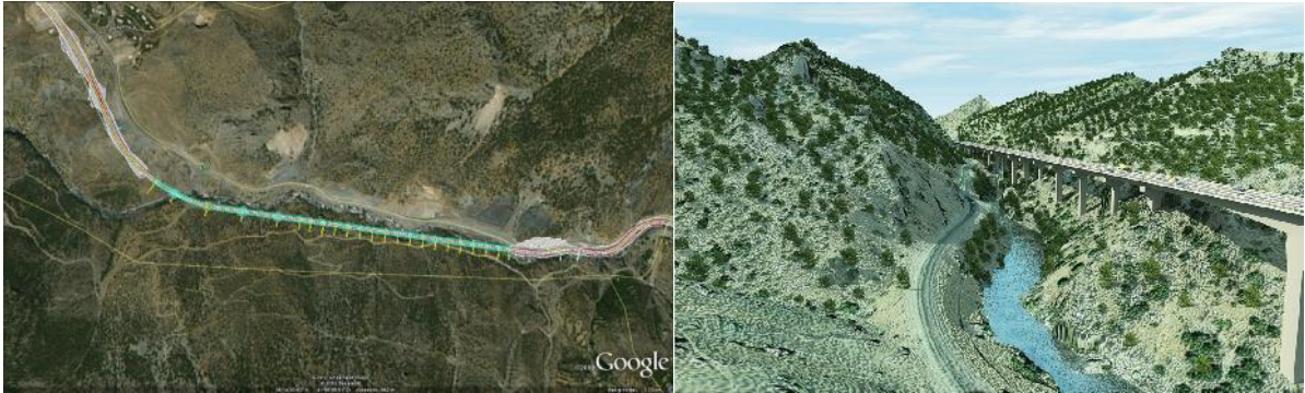
Figure 1. Satellite view and perspective view of the viaduct
